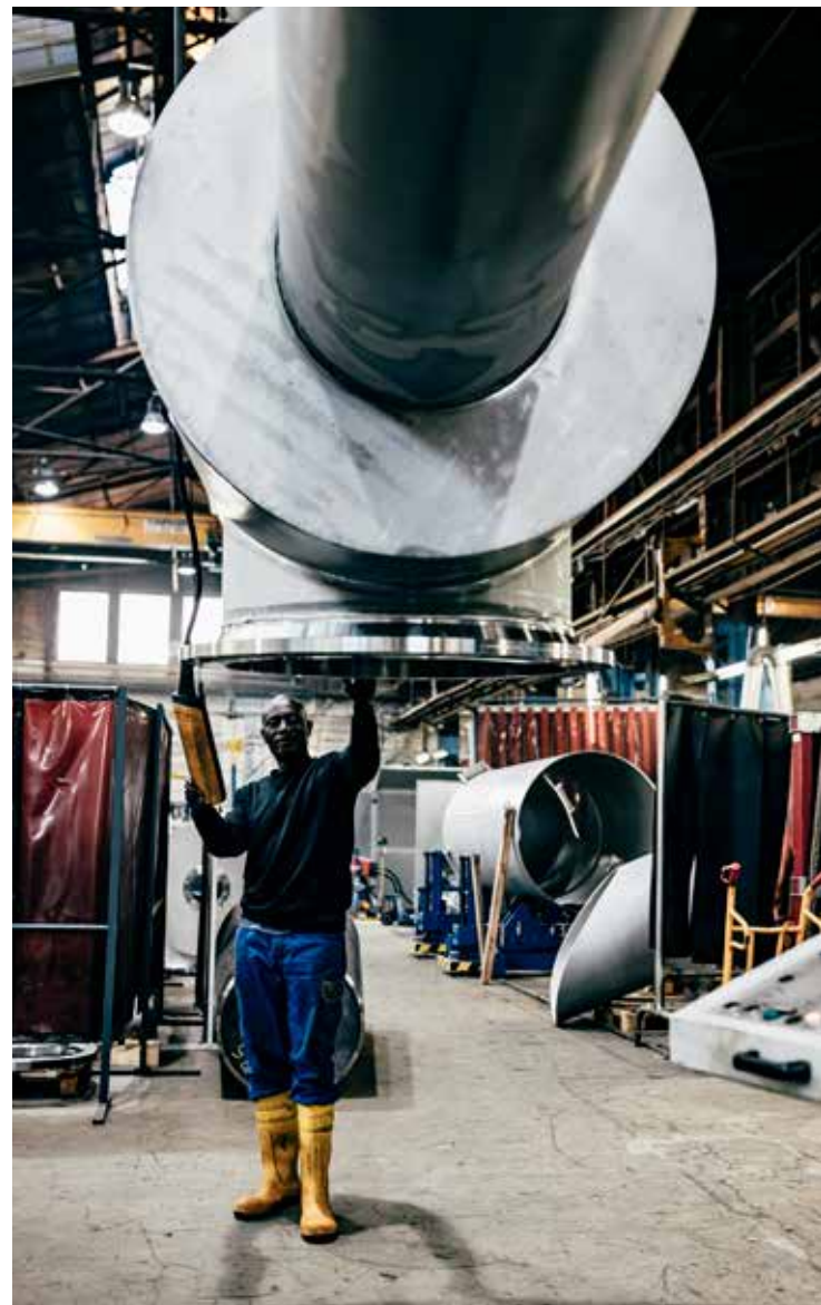
A steam jet ejector being made in Hanover
