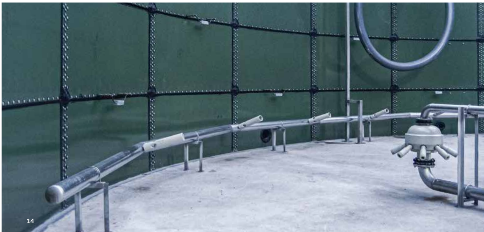
Liquid jet mixing nozzles for denitrification in an SBR plant
