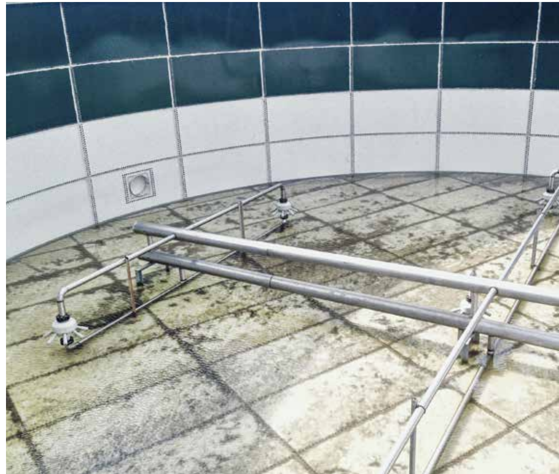
Seven-path ejectors in a 2 200 m 3 aeration tank in the cooking oil industry in Brazil
