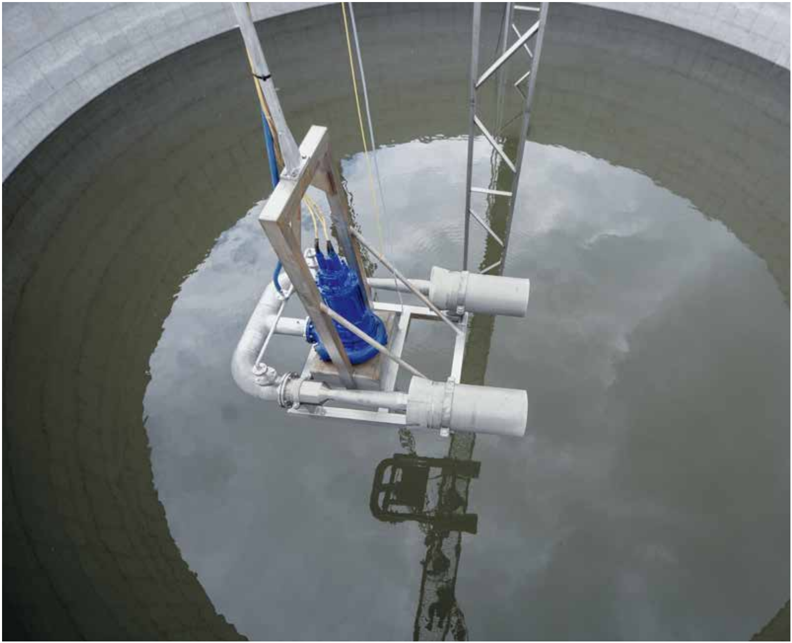
Mobile oxygen transfer system being submerged in the aeration tank of a company processing fruits and vegetables in Belgium. Installation was performed during plant operation by Westfalen AG. (Images © Westfalen AG, www.westfalen.com )
